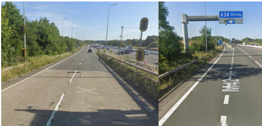
Figure 33: M42 J4 Northbound On Slip and Southbound Off Slip
